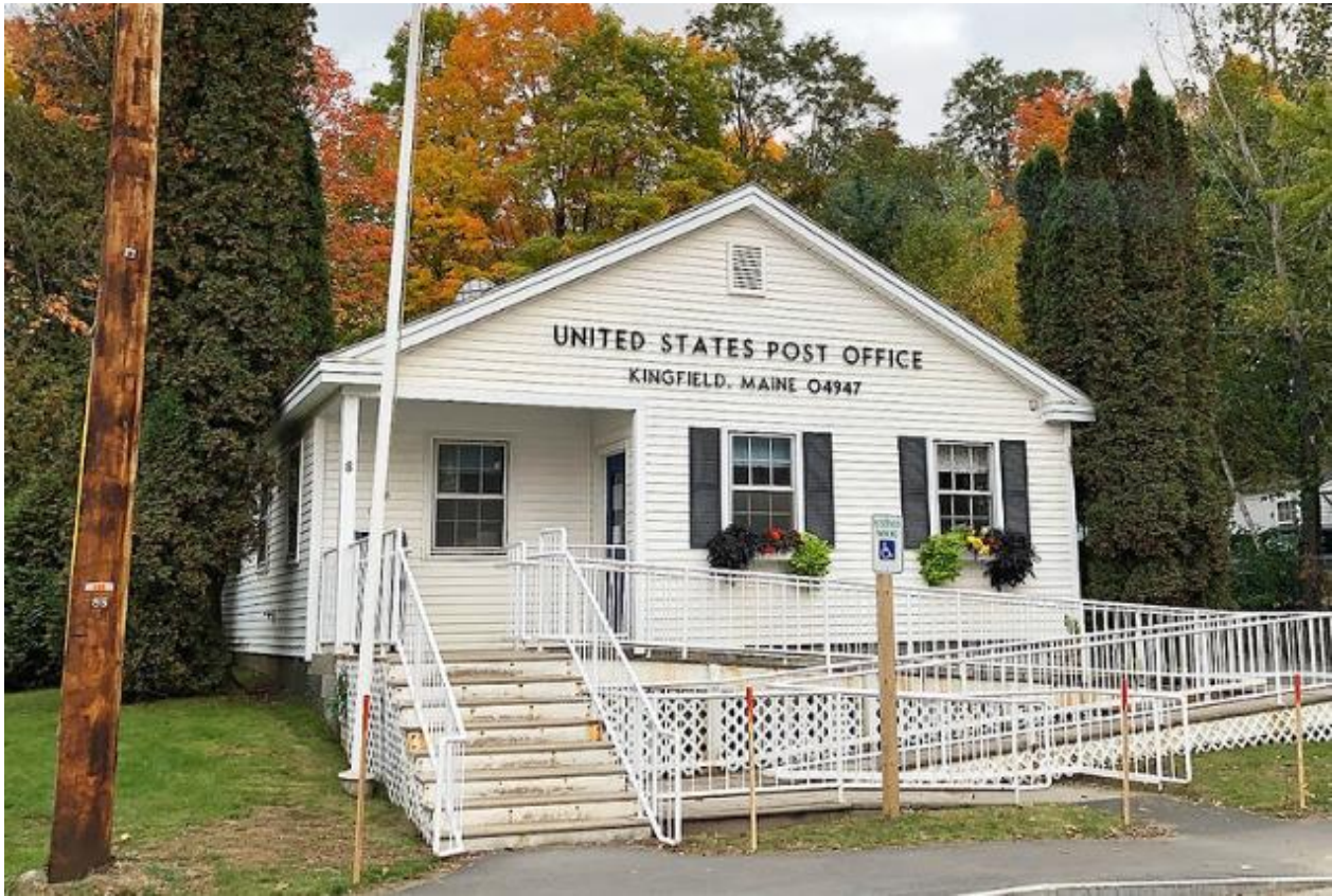
Kingfield, Maine Main Post Office
